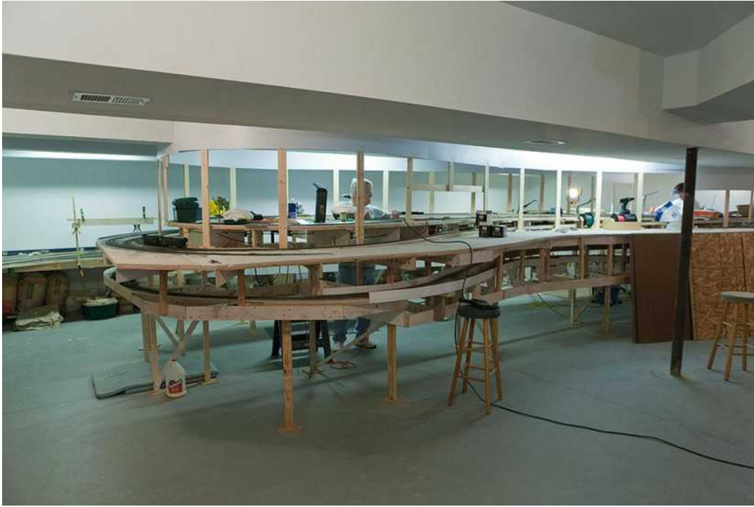
Vincent laying a small yard at the north end of the Fillmore Heights operators aisle.
